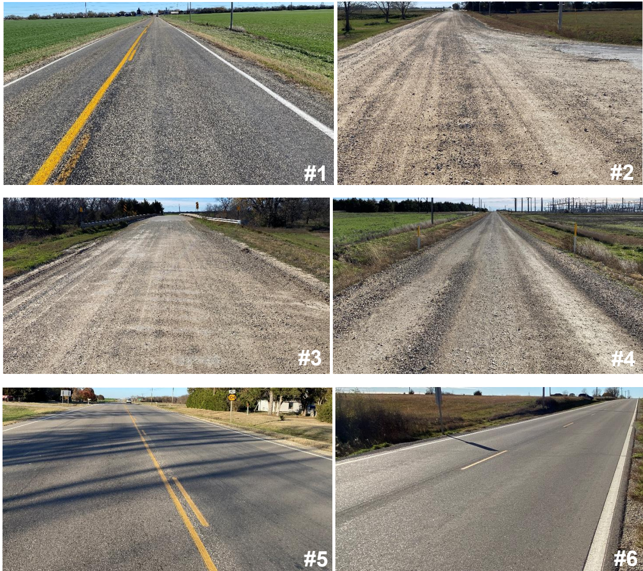
Figure 2 – Surface Condition Photos
